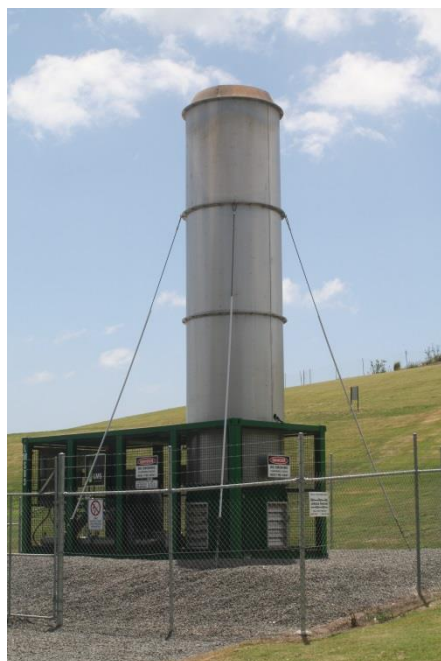
Fig 13: Flaring of Methane Gas
